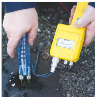
MOISTURE PROBE TESTING
